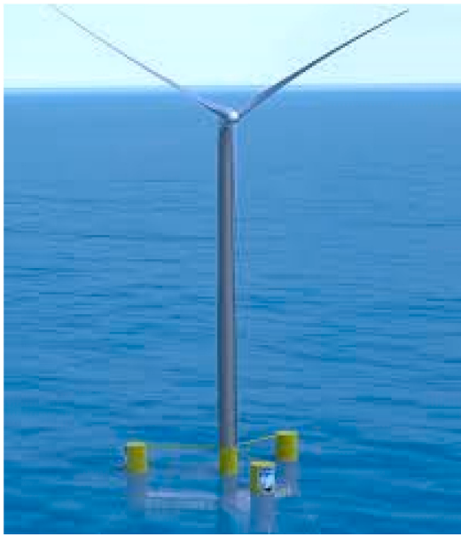
Fig. 3. The semi submersible floating wind turbine with nominal power of 15 MW [37].
