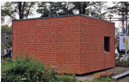
Facade panels for pumping station in the Amsterdam water supply dunes
