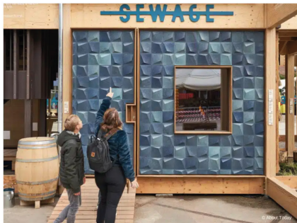
Facade panels with residual streams from water authorities
