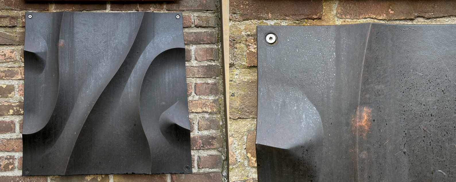
Figure 36. UV discoloration of the panels
