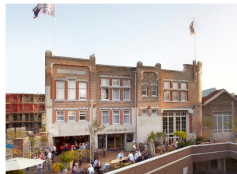
Figure 72 De Hallen after transformation (Acram, 2015)
