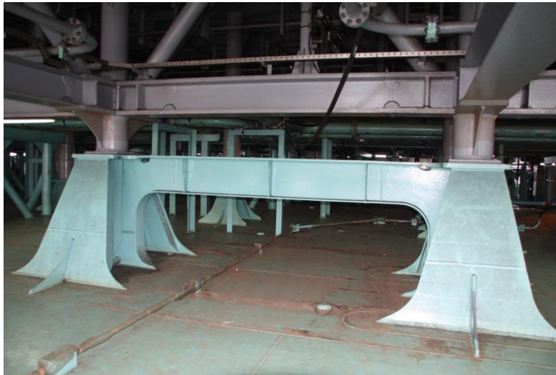
Figure 9 - Topsides connection with the deck
