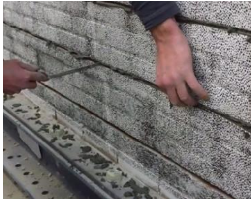
Figure 2.22: Execution of the bed-joint reinforcement technique (Licciardello et al., 2021 )
