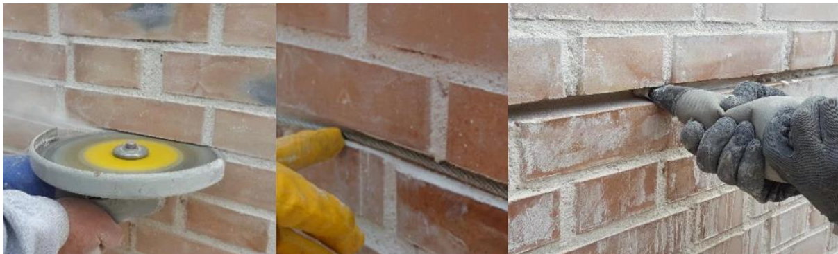
Figure 1.4: Application procedure bed-joint reinforced repointing (Corradi et al., 2020 )
