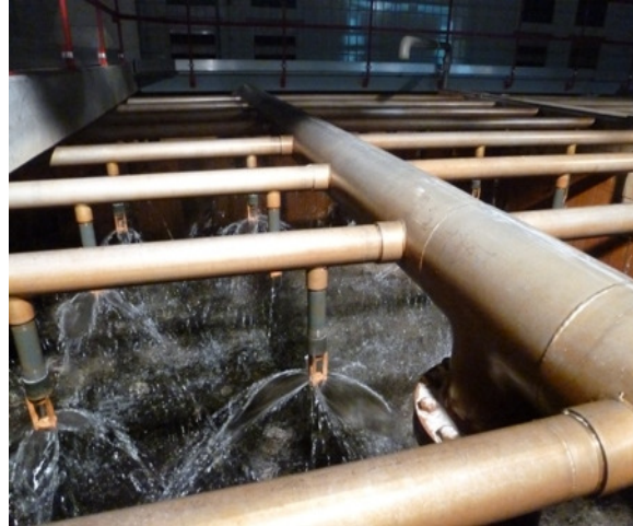
Figure 36: Spraying aeration on top of marble filter bed at Hoenderloo pumping station
