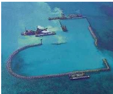
Figure 0-4 Construction of the initial stages of the artificial island
