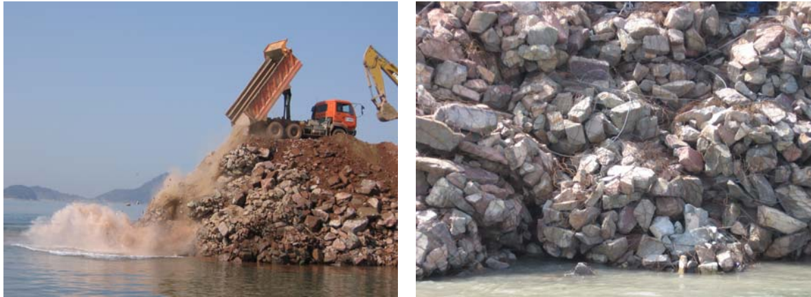
Figure 1.7: Dumping of gabions and settled gabions
