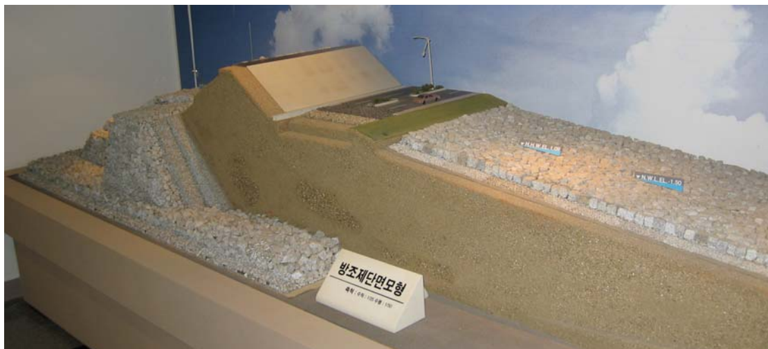
Figure 6.1: Model of the cross section of the Saemangeum dam
