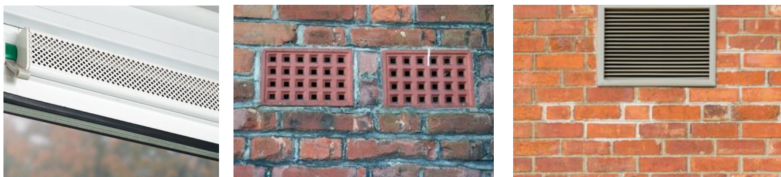
Figure 12: Trickle Vent (left), Air Brick (middle), Ventilation Grill (right)
