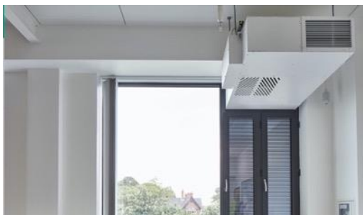
Figure 16: NVHR 1100 system by BreathingBuildings ( Breathing Buildings , 2020)
