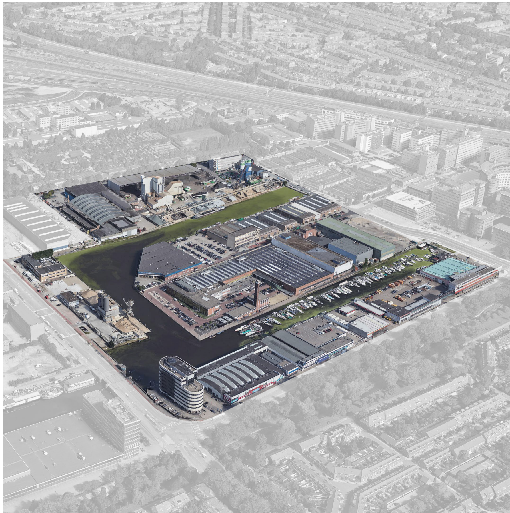
Aerial view Binckhaven
