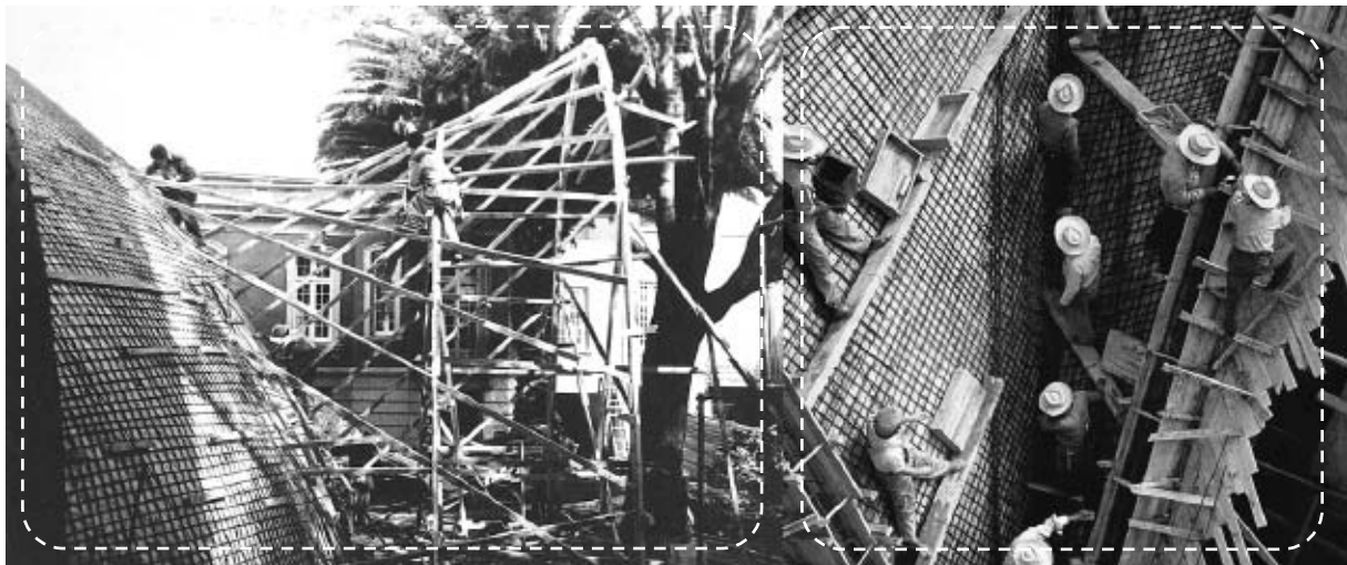
Figure 4: formwork construction by Felix Candela 2
