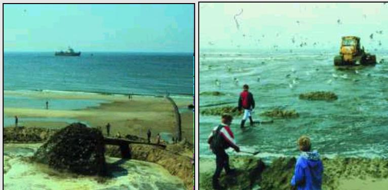
Figure 3.2 Beach nourishment operations off the island of Texel. Sand is transported through a pipeline onto the beach (a), after which it is spread by bulldozers (b), source: RIKZ
