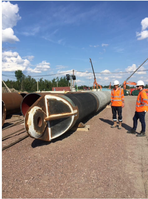
Figure 3.2: Pull head of 48' pipeline
