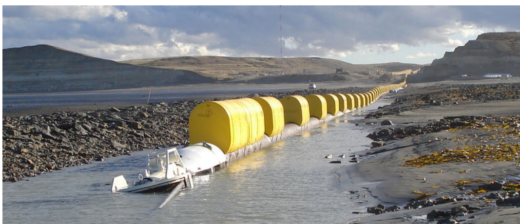
Figure 1.1: Pipeline pull-out operation in Magellan, Argentina
