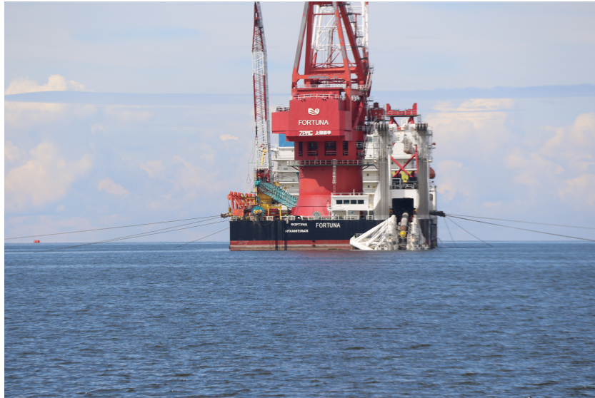
Figure 1.2: Pull-in operation from pipelay vessel stinger in Kurgalsky, Russia
