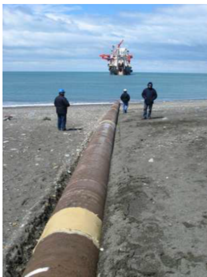
Figure 1.3: Pull-out operation from shore in Magellan, Argentina
