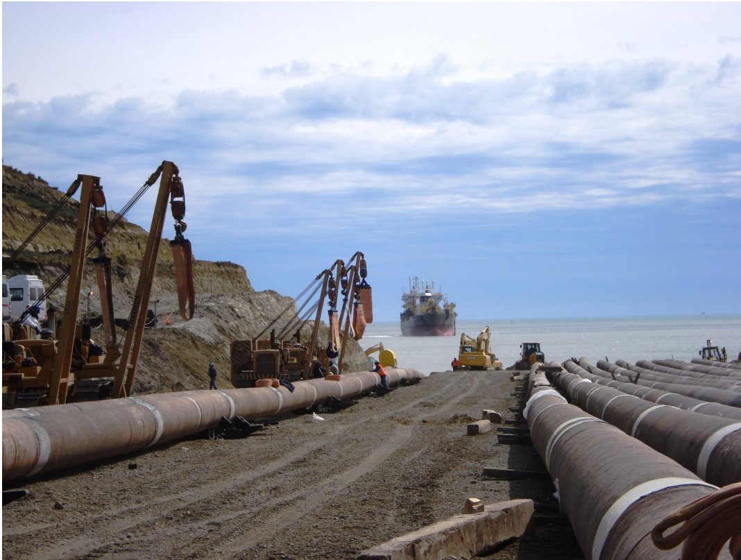
Figure 1.4: Example of a firing lane (l) and stringing yard (r) in Magellan, Argentina
