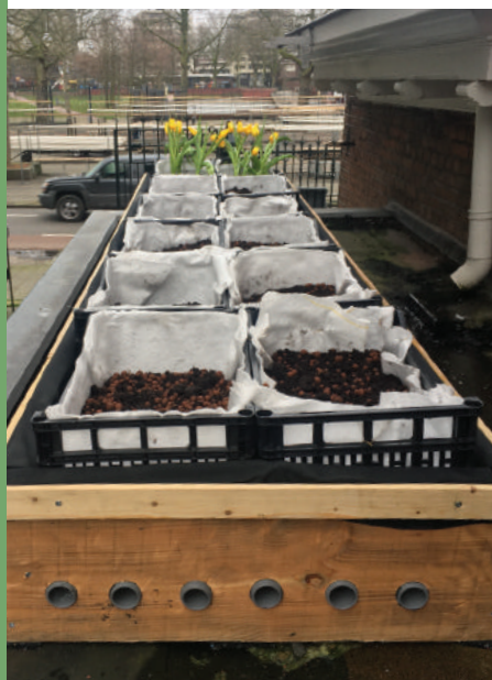
DIY green roof, made from used market crates
