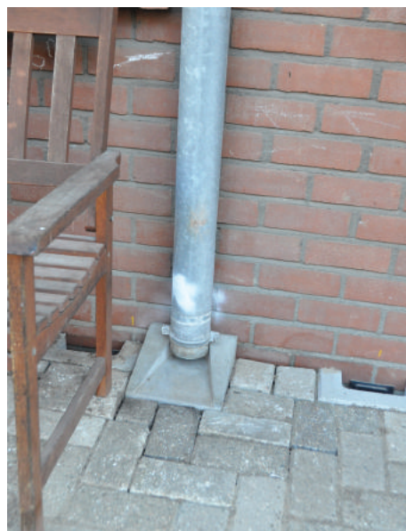
Disconnected drainpipes
