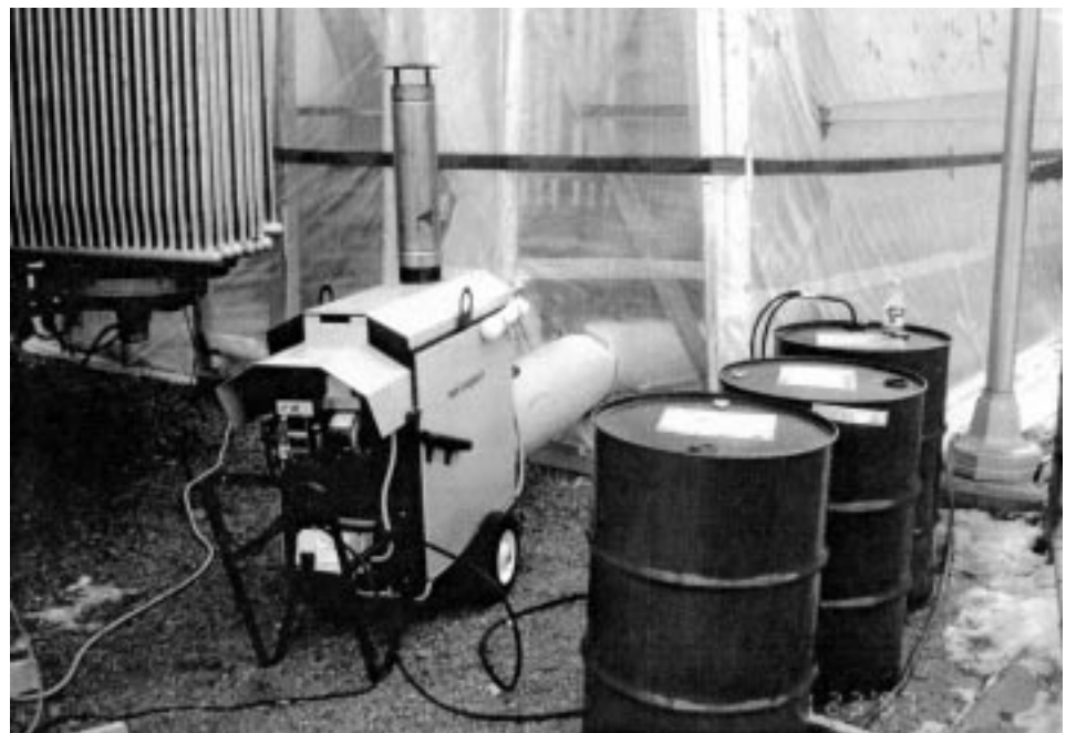
Figure 6. Space heater used to heat a plastic enclosure, Gavins Point project, Yankton, SD
