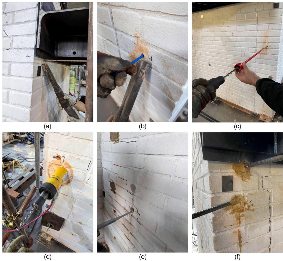
Fig. 4. Retrofitting steps: (a) hole drilling, (b) compressed air cleaning, (c) twisted bar installation, (d) twisted bar removal, (e) adhesive injection, (f) rebar installation.
