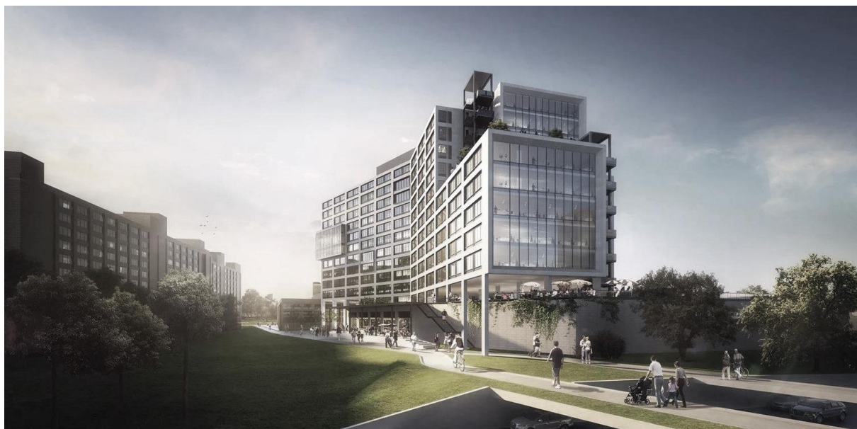
Figure 14: Carboncure technology used in a completed project in Atlanta, Georgia (Source: https://www.carboncure.com/case-studies/2018/5/26/725-ponce )
