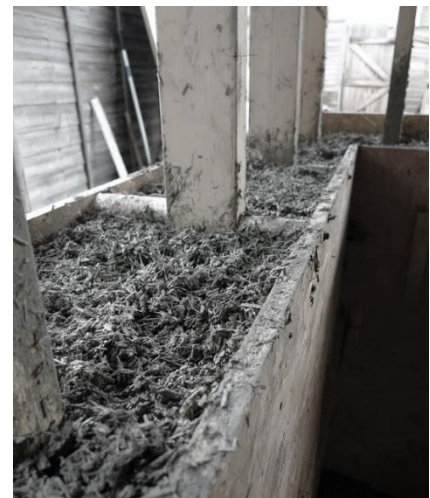
Figure 12: Hempcrete cast-in-situ method (Stanwix & Sparrow, 2014)
