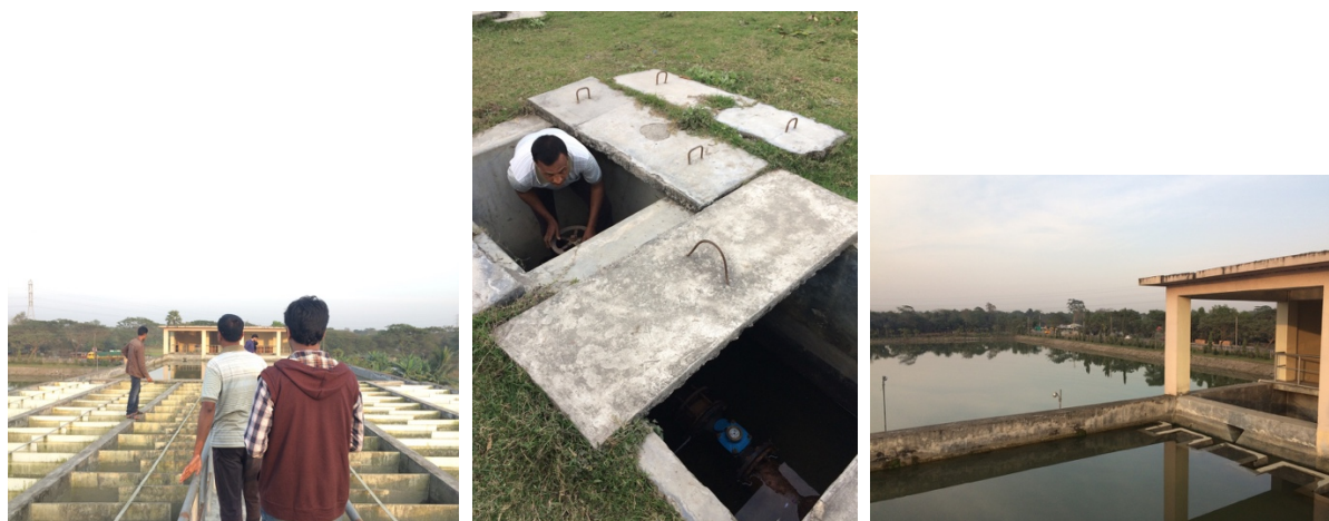
Figure 23: Water supply treatment plant for governmental institutions
