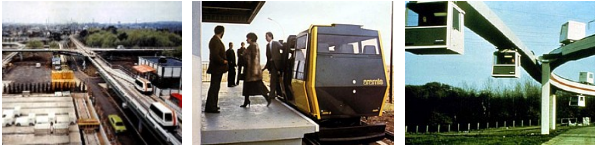
Figure 2-1: Left: CVS test facility Tokyo, center: Aramis test facility, right: Cabintaxi test facility (reprinted from Khammas 2017)
