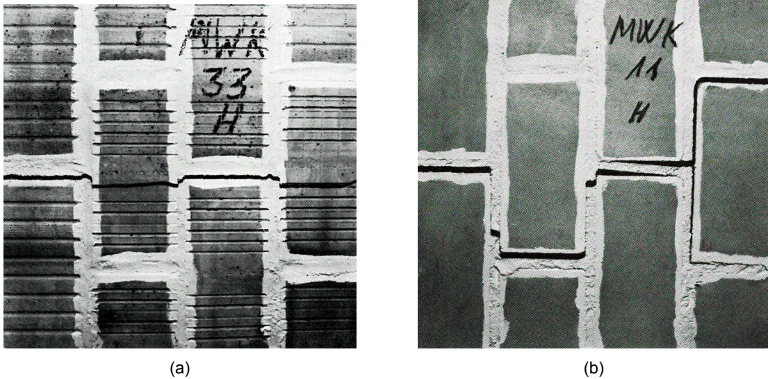
Figure 1.6: Modes of tension failure of masonry walls under direct tension (from [5]): (a) through type, (b) zigzag type
