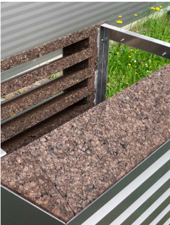
▲ Figure 54 - Cork applied in the Brockx
