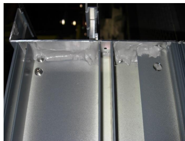
(a) The connection between the mullion and transoms with sealant, made by Scheldebouw (Contact nr. 1)(2020)
