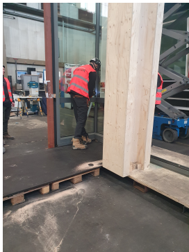
(c) Drilling holes in the framing on the inside
