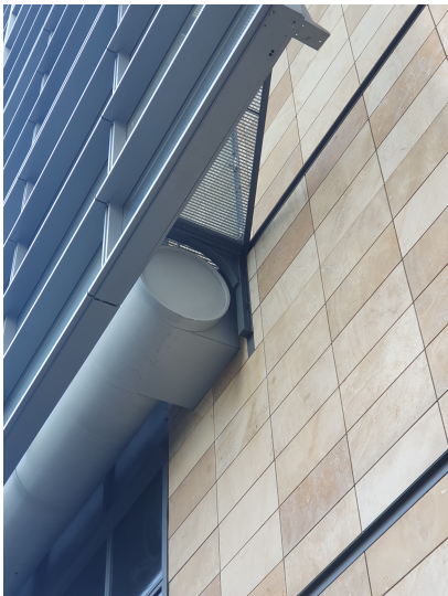
(d) Picture of Gallow brackets, walkways and tubing in the cavity of the refurbished facade of 1 Triton Square
