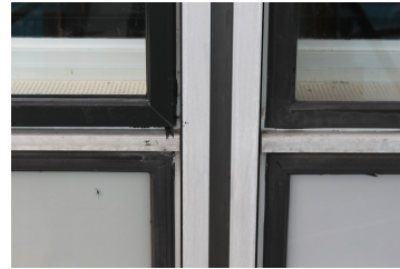
(b) Comparison of the refurbished and old facade, upper right is the old connection, upper left is the new connection. Made by Scheldebouw (2020)
