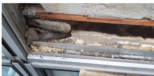
(a) The aluminium profile after the glazing was removed
