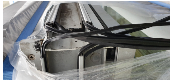
(b) Replaced EPDM gaskets
