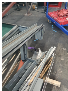
(c) Some more leftover debris that was left over from the dismantling. The sealant that was cut off the windows is still visible and the aluminium elements that were cut up.
