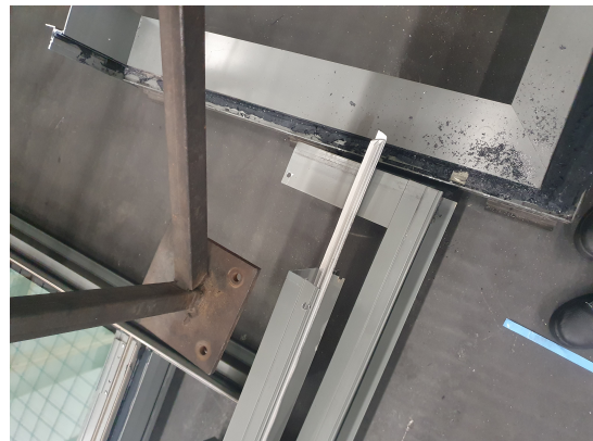
(d) The leftover sealant from the glazing can be seen in the groove.
