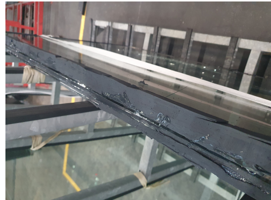
(b) In this image the leftover sealant on the glazing can be seen. It was cut from the aluminium element in order to take out the glazing from the element. The glass was slightly damaged in this process.
