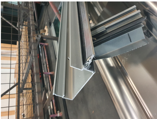
(c) Aluminium profiles were cut for them to be removed. This element in particular was the top or bottom mullion where the elements were connected to each other.
