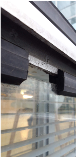
(b) The view of the EPDM gaskets and the status of the framing in the Koningskade
