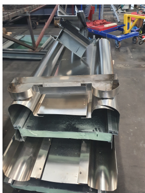
(a) Aluminium elements with insulation in them, were cut down for them to be removed.
