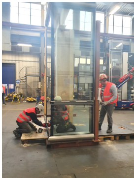
(f) Cutting the sealant of the windows
