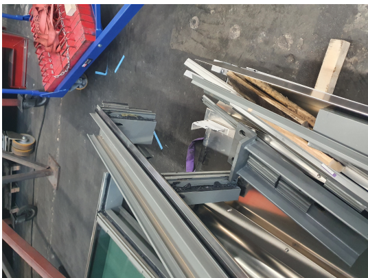
(e) Some more leftover debris that was left over from the dismantling. The sealant that was cut off the windows is still visible and the aluminium elements that were cut up.
