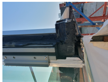
(b) One of the vertical cut profiles, remaining of the sealant can be seen, also the mechanical strips that keep in the glazing.
