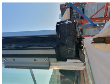
(b) One of the vertical cut profiles, remaining of the sealant can be seen, as well as the mechanical strips that keep in the glazing.
