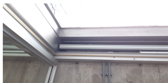
(b) The aluminium profile after the glazing was removed, from the inside
