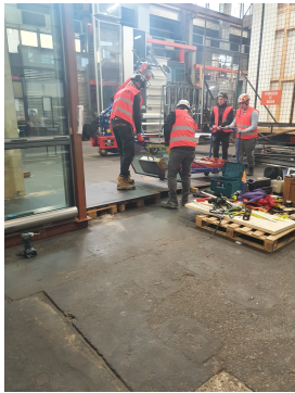
(l) The glazing taken out of the framing
