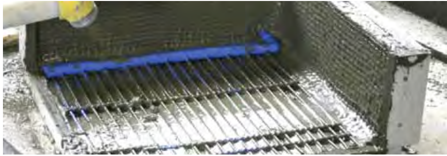
Figure 7.8 Inserting capillary elements into fibre reinforced concrete
