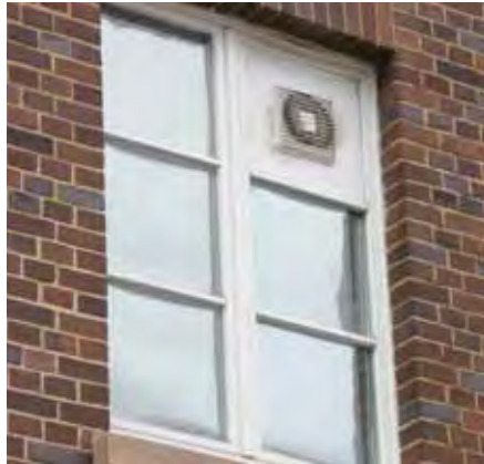
Figure 5.22: Built-in fans in a server room
