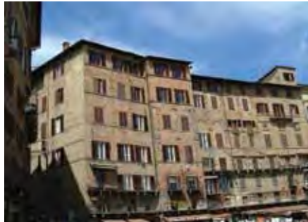
Figure 3.15: Low share of window area at the Piazza del Campo in Siena.
