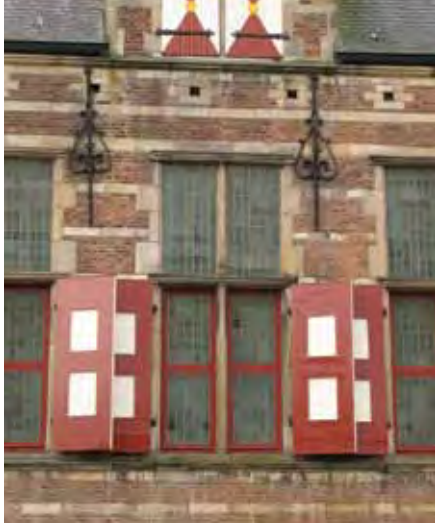
Figure 4.1: Dutch window; in early stages outfitted with folding shutters in the lower section to offer ventilation but provide rain tightness at the same time; and lead glazed window panes for lighting in the upper section.
