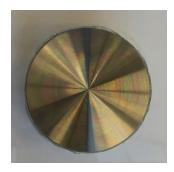
Figure 2.2: TSSA laminated connection as seen through the glass
