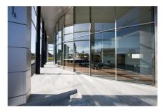
Figure 1.2: Linearly supported glass facade (Source: Forster Profile Systems)
