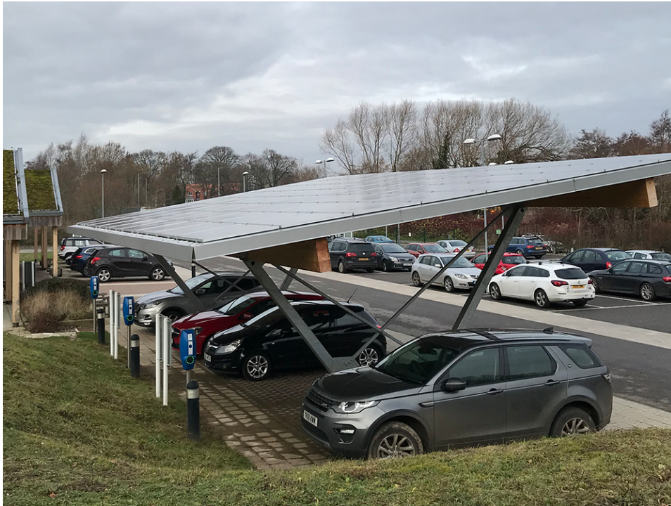
Figure 1.1: Example of a grid-connected solar carport used for EV charging [1]
