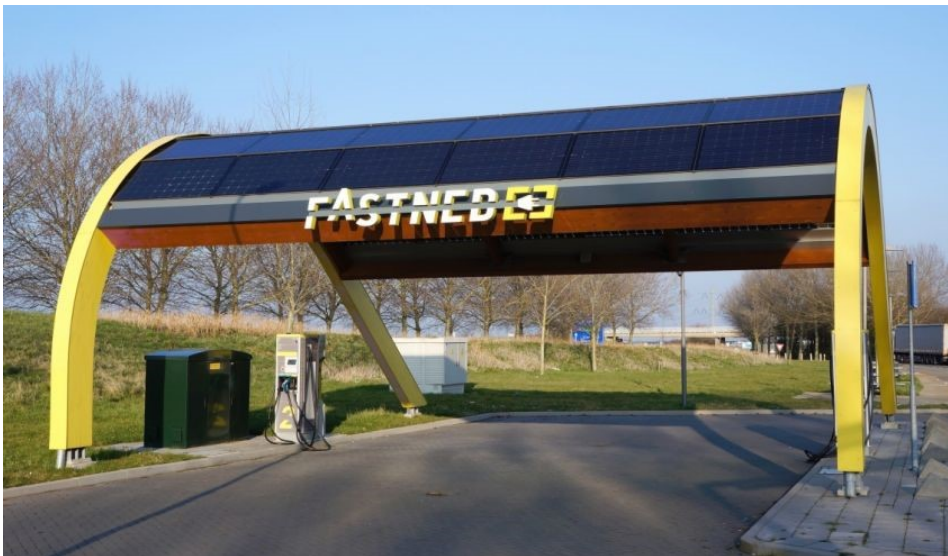
Figure 2.7: FastNed system installation [4]
