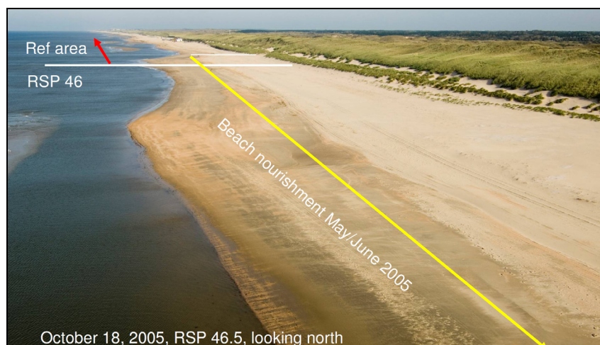
Figure 2-3 Beach nourishment done at Heemskerk in the year 2005
