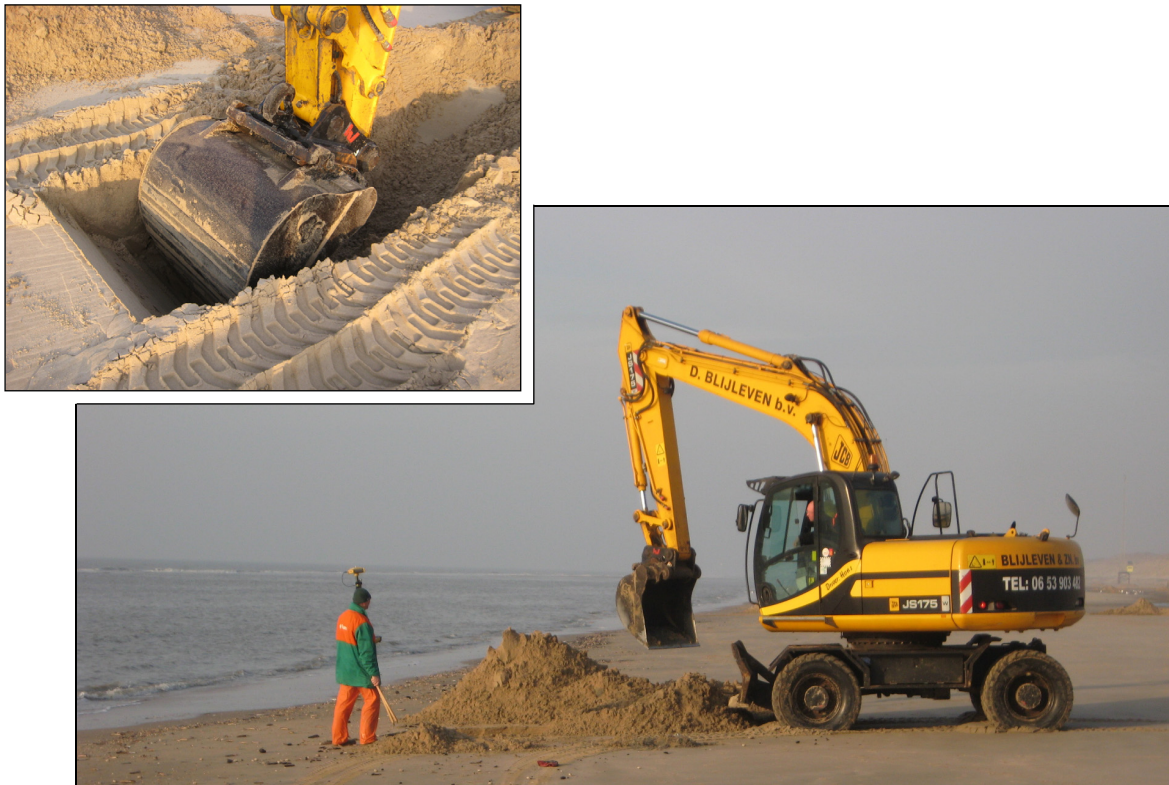
Figure 6-12 Removal of the vertical drainage tubes near Egmond aan Zee
