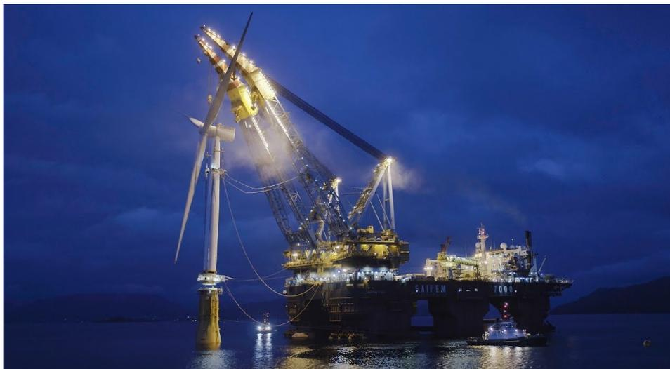
Figure 2.2: The Hywind Scotland wind farm under construction (Equinor, 2017).
