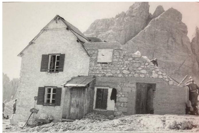
Renovation works in 1962. Source Zandonella Callegher
