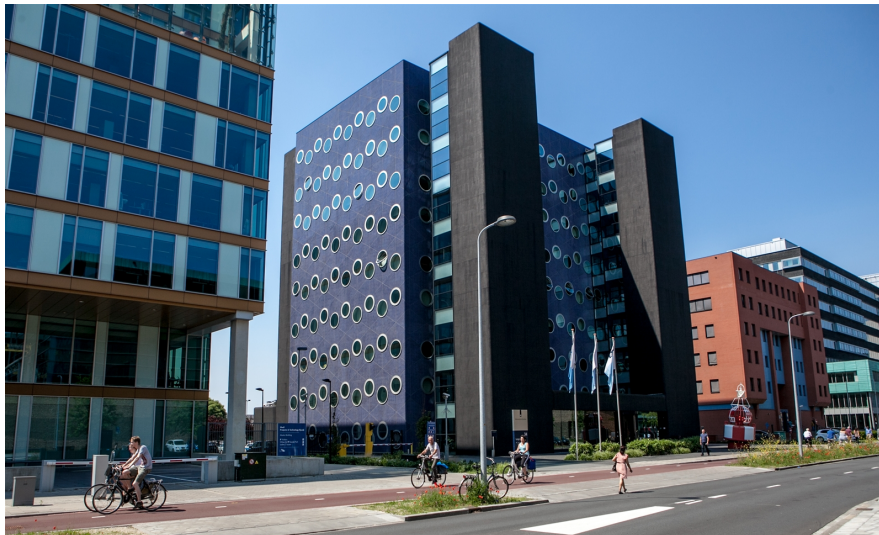
Figure 1-3: The Rijkswaterstaat Rijswijk Testbed
