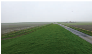
Fig. 46b: Secondary dike/ sleepy dike
