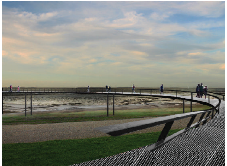
Fig. 102c: Metal loop giving a panorama view from the dike to the dynamic Wadden sea (10 years)
