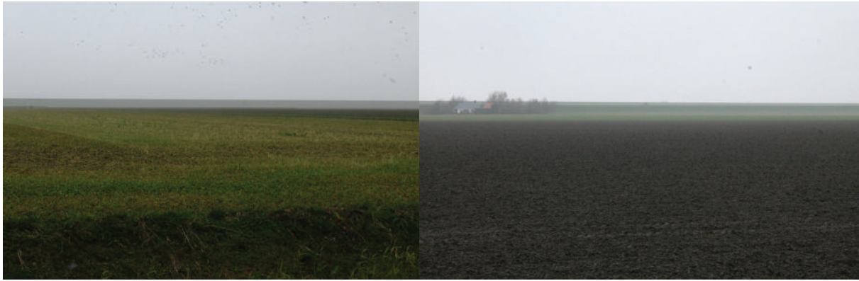
Fig. 5a: The sea dike as endless wall enclosing large plots of fresh water production land ; seen from the inside of the dike (Own library)
