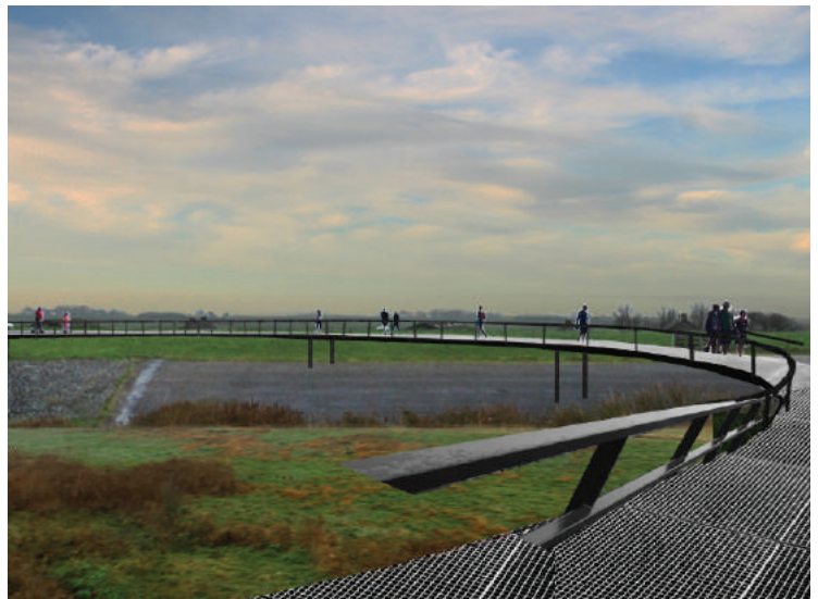
Fig. 102b: Metal loop giving a panorama view from the other side to the primary dike & main land behind (10 years)
