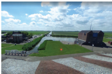
View from tiled dike to water basin, straight boezem and pumping station
