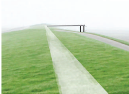
Fig. 102a: The metal loop as destination of the path on the primary dike
