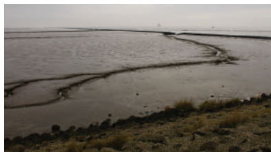
Fig. 43b: Current gullie, sedimentation and erosion
