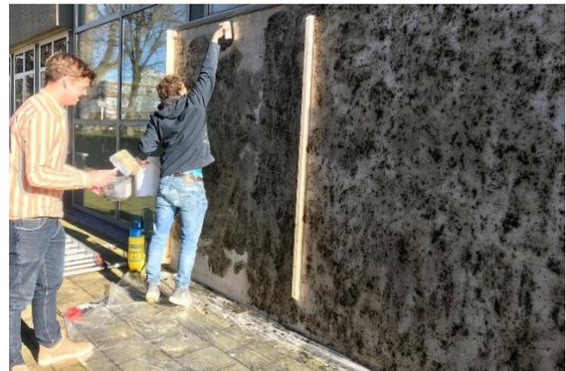
Figure 14. Photograph capturing Respyre team applying the moss mixture.
