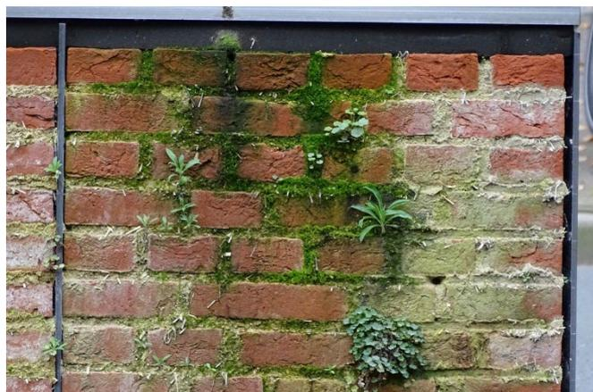
Figure 17. Photograph of the vivid plant growth on the mortar that appeared to contaminate the water. Image by K. Molder.
