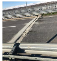
Figure 2. Joint movement and joint pounding [18]
