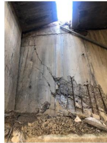
Figure 6. Concrete Spalling [18]
