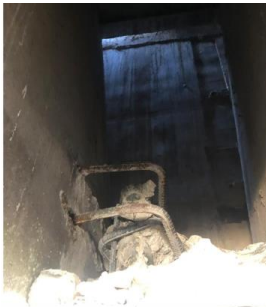
Figure 4. Shear Key Failure [18]
