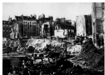
1.06 Demolitions planned by Haussmann to create Avenue de l'Opéra. Charles Marville, Between rue
