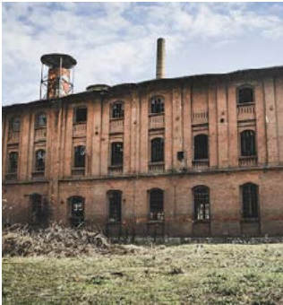
Delicate Brick Facade
