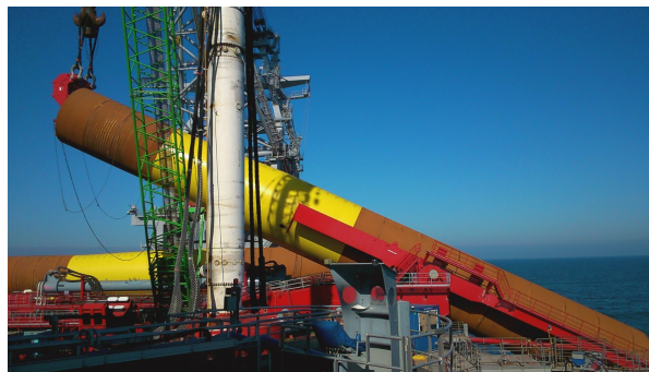
Figure 1.3: Upending monopile (2016, IHC)
