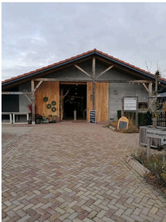
Fig. 3. The re-used farm building of Mouthoeve, Source: First author (2020).
