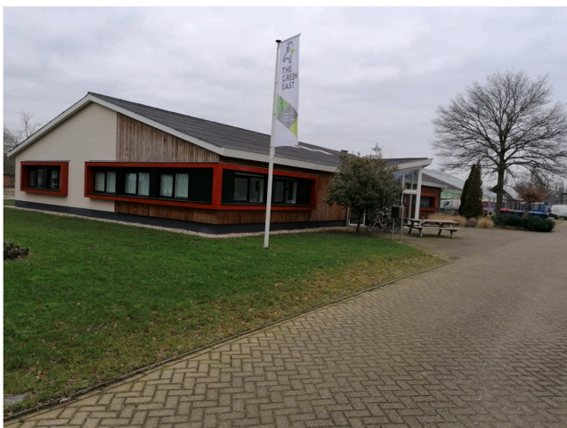
Fig. 6. The re-used farm building of The Green East, Source: First author (2021).
