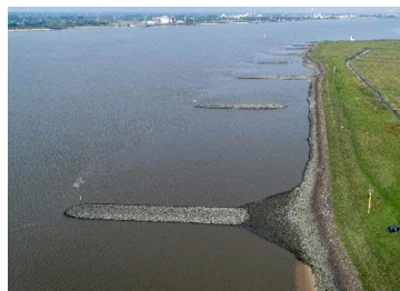
Figure 1.1: River groynes perpendicular along the Lower Elbe Estuary in Germany (Melling et al., 2020)
