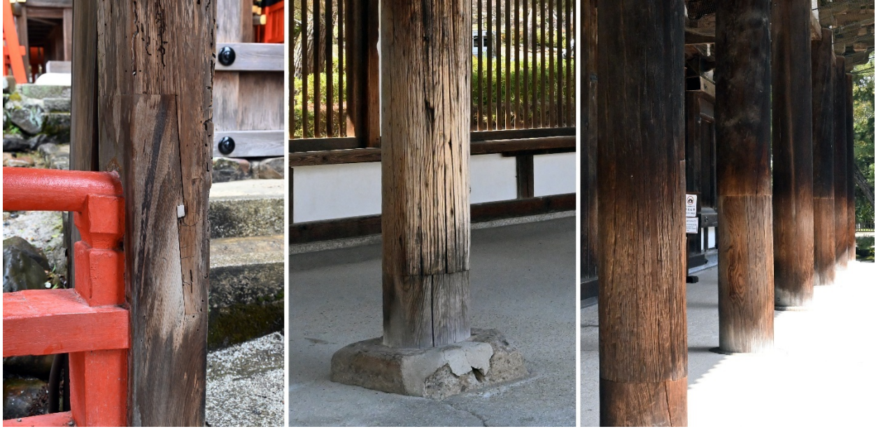
Figure 3.13: Minor maintenance: Components partly replace (Taken onsite)
