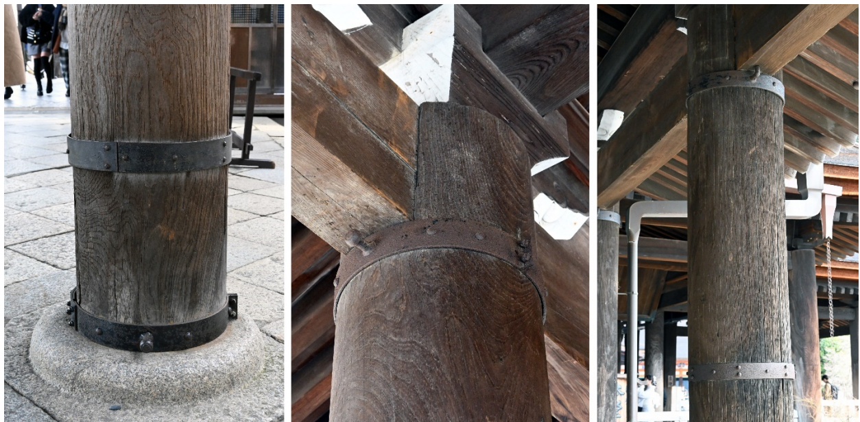
Figure 3.12: Minor maintenance: Metal fasteners (Taken onsite)
