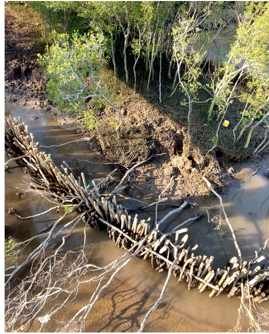
Figure A.6: Cliff formation indicating erosion behind bamboo fence
