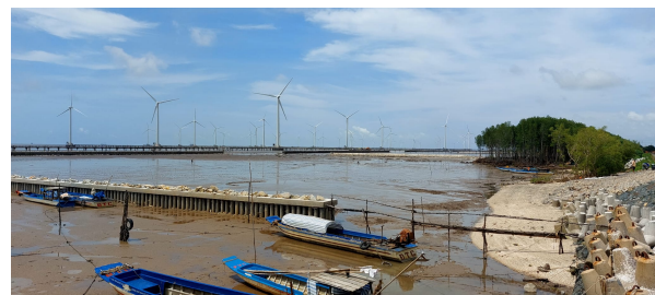
Figure A.4: Newly build pile rock breakwater at Bạc Liêu border
