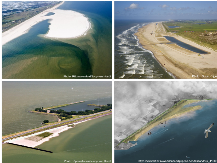
Figure 1.1: Aerial photographs of four nature-based sandy solutions in the Netherlands: a) the Sand Engine, b) the Hondsbossche Dunes, c) the Houtrib Dyke, and d) the Prins Hendrik sand dyke (artist impression).
