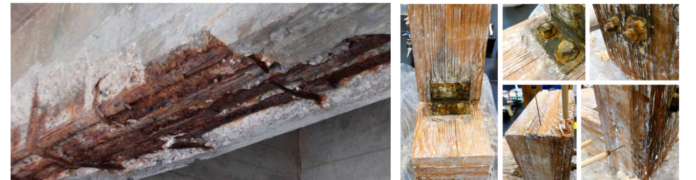
To the left, Deterioration of concrete due to corrosion ( structuralguide.com ). To the right: images of a test for a CLT connection under wet conditions for a prolonged period of time (Cappellazzi et. al, 2020).
