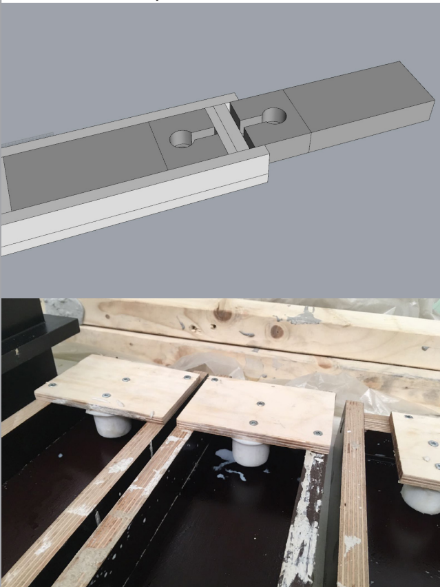
Figure 19: Formwork Concrete Segments (Peter Eigenraam, 2018)
