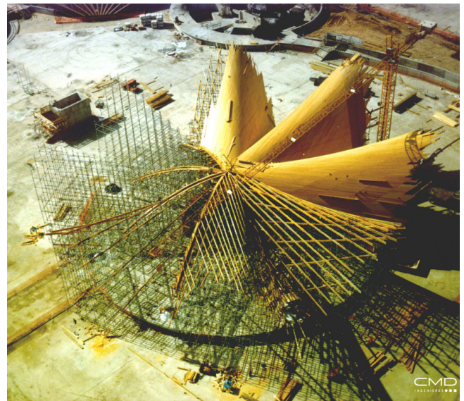
Figure 11: Temporary structure underneath the shell (CompetitionLine, 2012)
