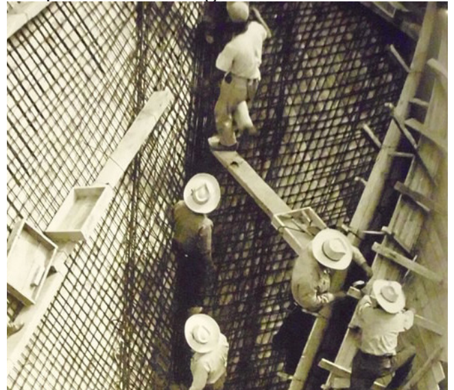
Figure 13: Construction the Los Manantiales, shell structure (skyscrapercity, 1958)
