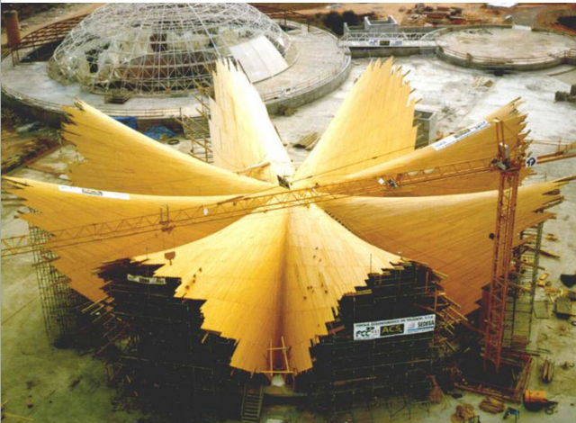
Figure 12: Formwork on the structure (Domingo et al, 2004, p. 1148)
