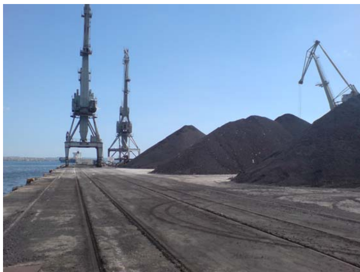
Figure 266 Rail tracks at the eastern part of Pier 5
