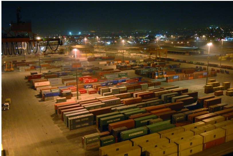
Figure 30 Night view of the storage area of the C.T.
