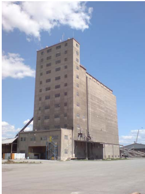
Figure 277 The Silo located at Pier 4
