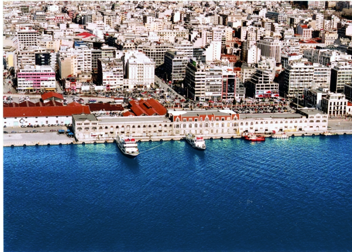
Figure 47 Aerial view of the main building of the P.T. [ThPA SA]
