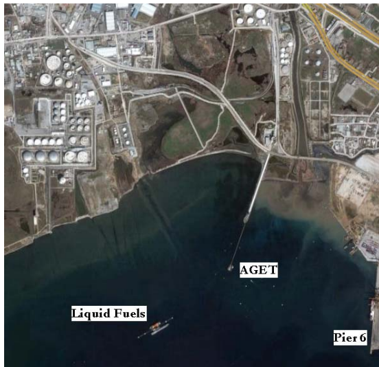
Figure 49 Satellite picture of the area west of Pier 6
