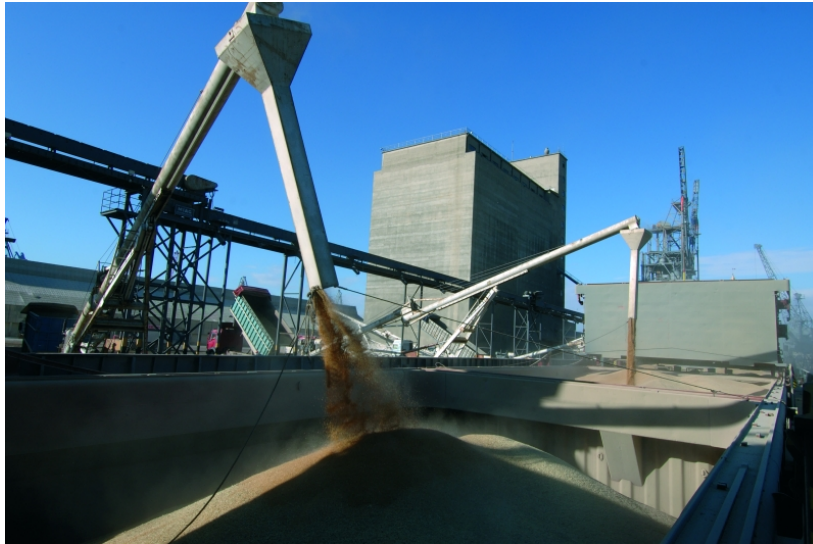
Figure 288 Loading mechanism serving the Silo at Pier 4 [ThPA SA]
