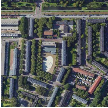
Figure 2.58 Aerial view of Heeswijkplein Source: Google earth
