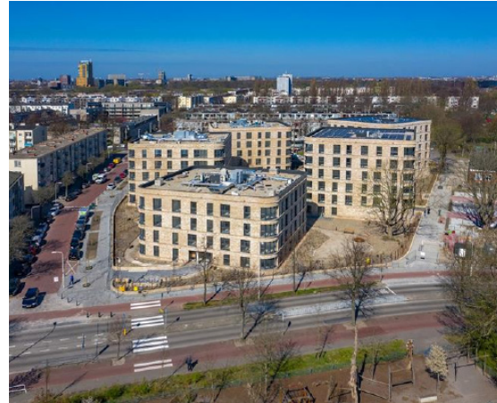
Figure 3.8 Example of replacement (n.d) Source: https://www.arcadewonen.nl/objecten/westhovenplein/
