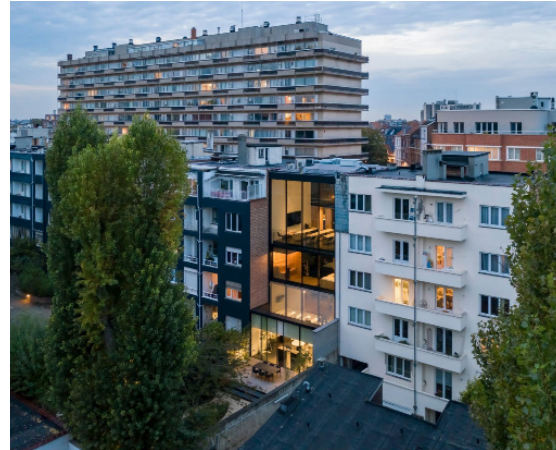
Figure 3.4 Example of infill (z.d). Source: https://archello.com/nl/news/infill-project-in-brussels-uses-glass-to-create-intriguing-spatial-transitions
