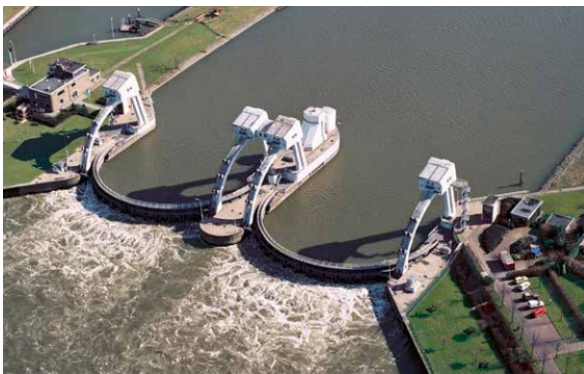
Figure 1.1: Top view of weir Hagestein (Rijkswaterstaat, 2020 )
