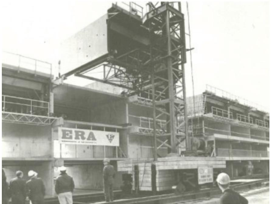
*Figure 17 ERA system under construction. Steel casting module lifted by tower crane.*
