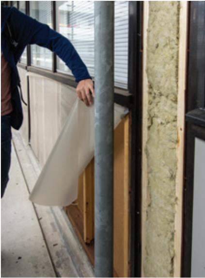
*Figure 16 Wooden facade under thermal renovation (2016). Additional layers of mineral wool inserted for insulation.*
