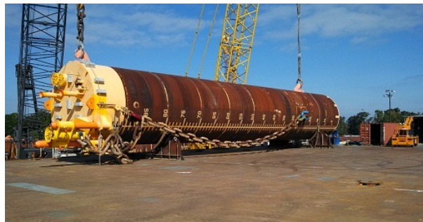
Figure 2.8: Suction pile [5]
