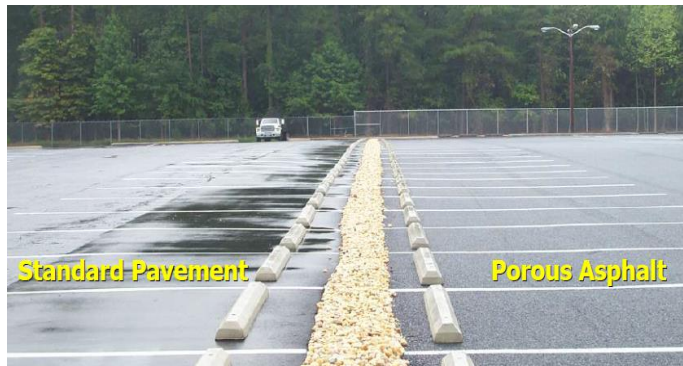
Figure 1.1: Water draining ability of porous asphalt [6].
