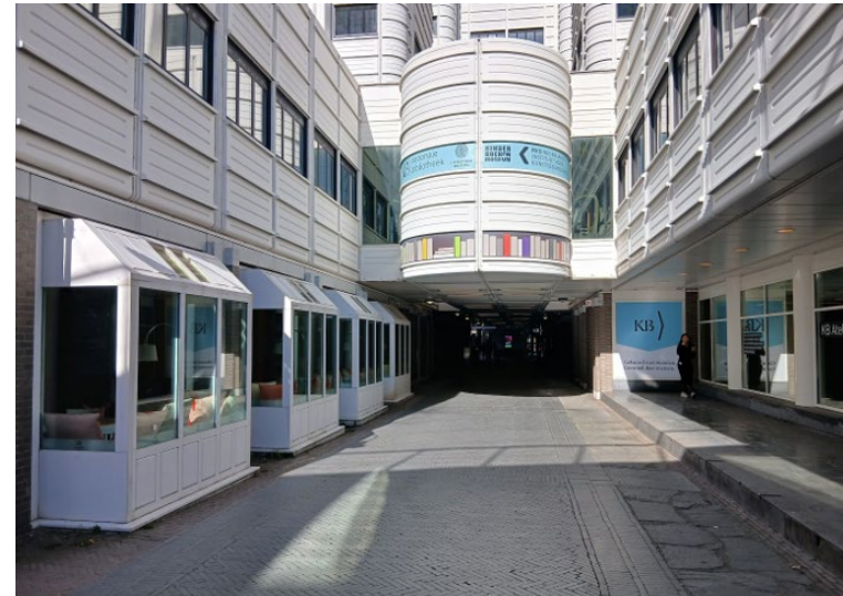
Figure 29: Narrow entrance towards the entrance
