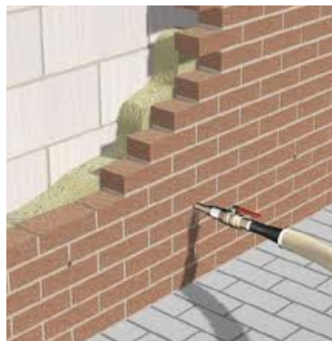
Figure 3.18: Illustration of cavity insulation being added (Ritsema, sd)
