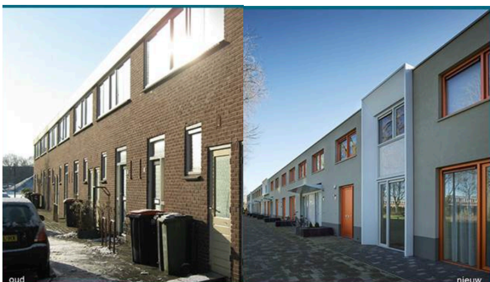
Figure 3.21: Added façade layers to improve the insulation (Milieu Centraal, 2021)
